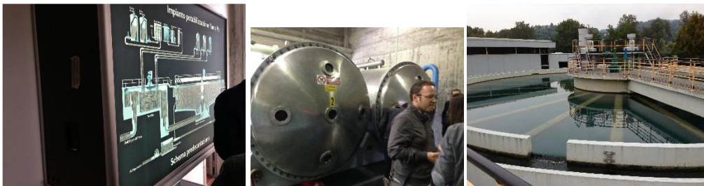
Figure 5: SMAT water treatment facility
